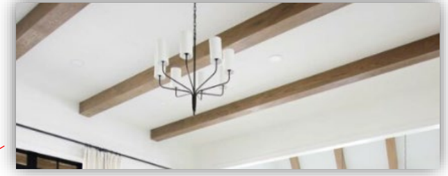
8" STAIN GRADE PINE BEAMS INSIDE TRAY
