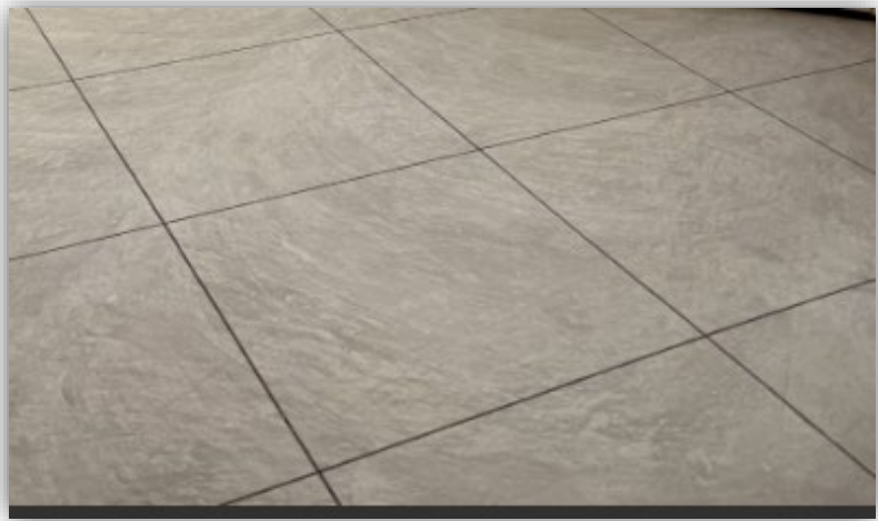
Porch concrete cut in decorative diagonal pattern
