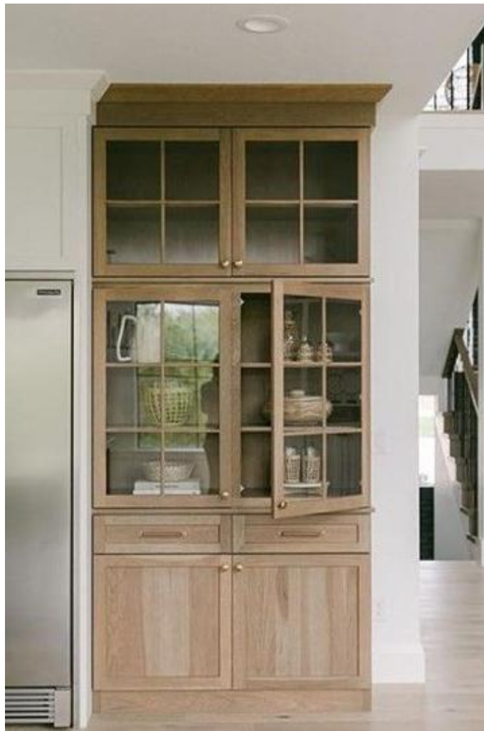
CABINET TOWER Cabinet tower with 4-pane glass fronts. LED tape lighting under fixed shelves and puck light in top uppers.
