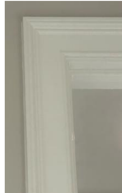
STANDARD WINDOW & DOOR CASING
